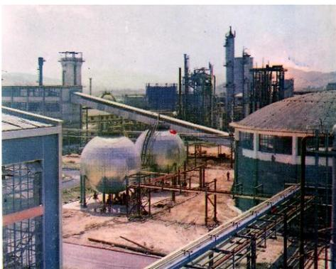
Figure 9.5 In this factory, nitrogen gas and hydrogen gas is combined to form ammonia, a key fertilizer for farmers.
